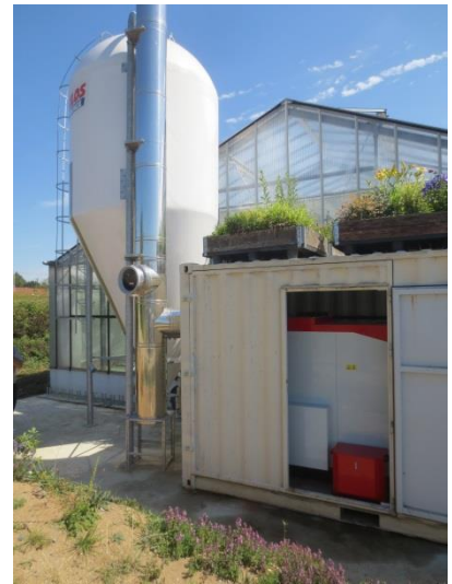
Chaudière Gilles – Centre horticole du RATHO – fourniture Agronerger
